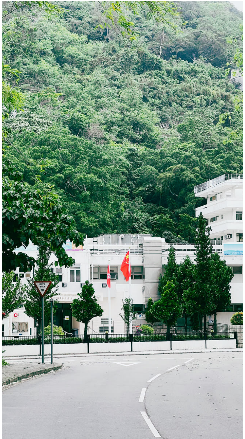
The façade of the Duchess of Kent Children's Hospital, as seen from the intersection of Sha Wan and Sandy Bay Road.
